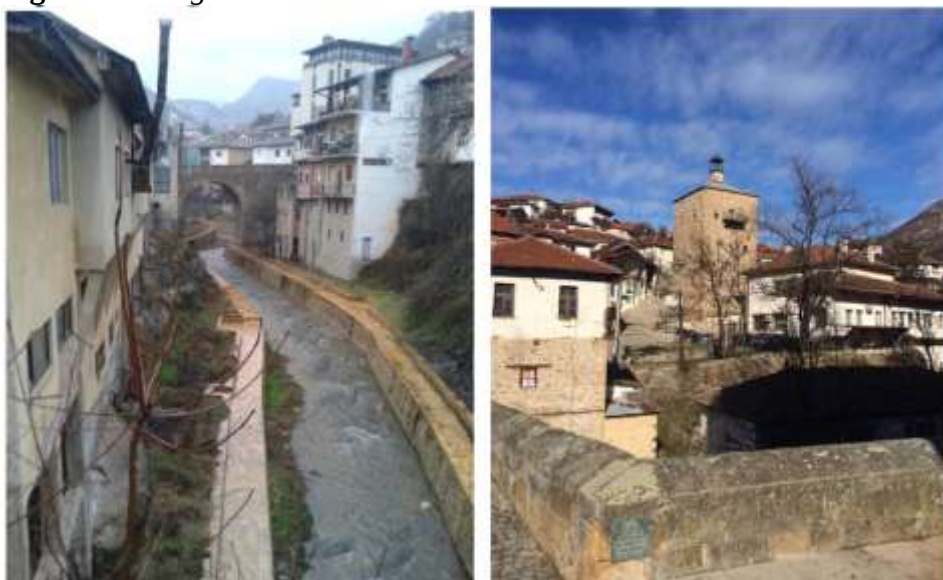
Figure 8: Bridges in Kratovo
